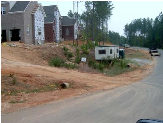
**BAD:** Either no stone has been placed, or it has worn down. This entrance lets sediment offsite and is messy during wet conditions. Sediment going onto the roads can cause the site to be in violation.
