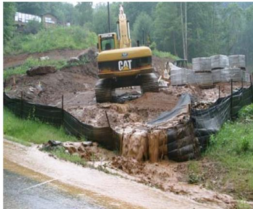
**BAD:** Silt fence is down and not attached to the post. It allows sediment off the site. Silt fence should not go down contours letting sediment and water to concentrate in one spot. This causes extra stress to the fence and causes failure. It is best to let the silt fence go across contours to allow flows not to focus on one spot.
